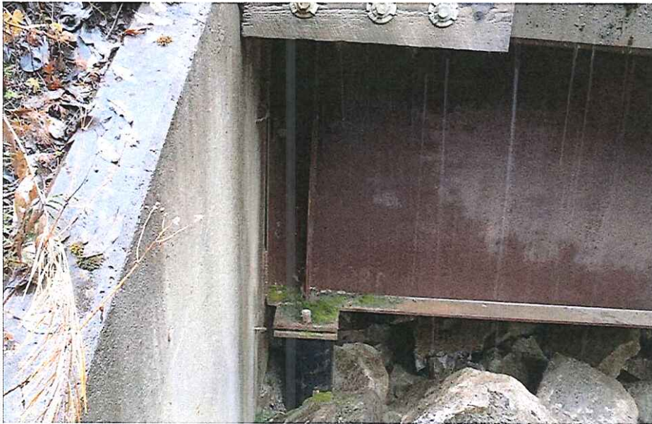
CK2306 Right Abutment Bearing
