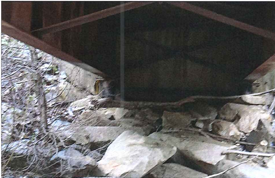
CK2306 Left Abutment
