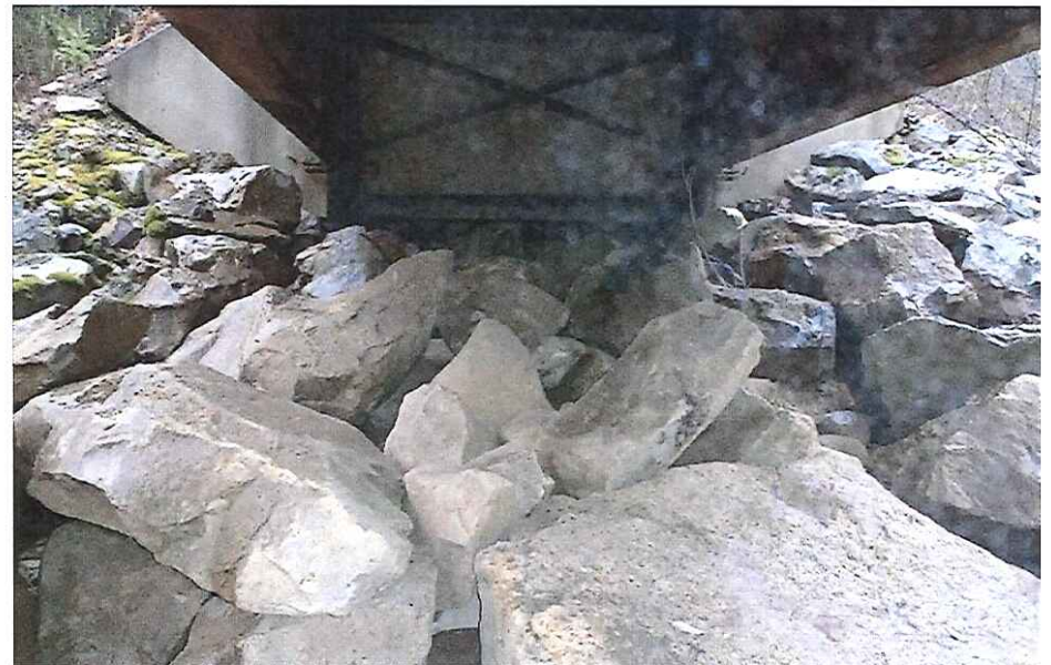
CK2306 Right Abutment
